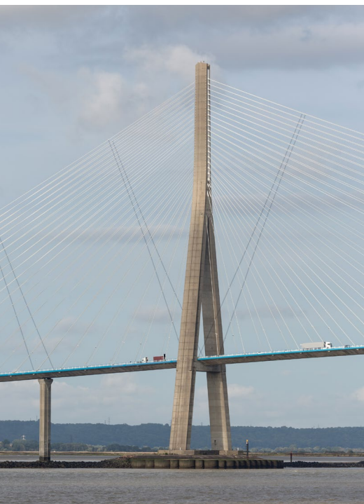
Drones can inspect infrastructure in places that are too dangerous for humans.
