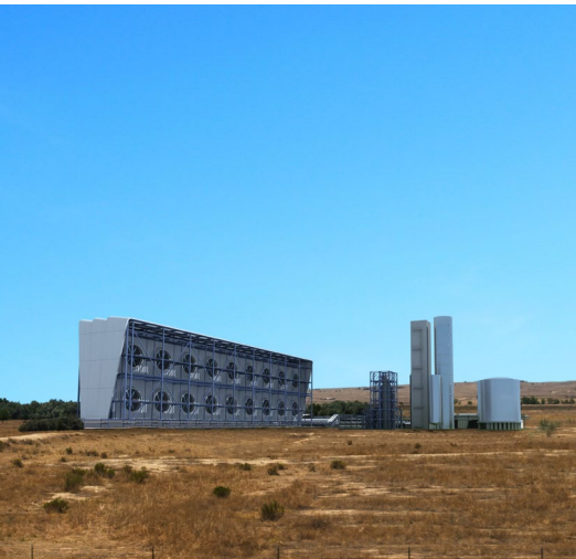
The world's largest Direct Air Capture (DAC) and sequestration facility.
